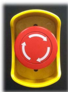
Figure 2-1: EMO Button Near Circuit Breaker Panel
